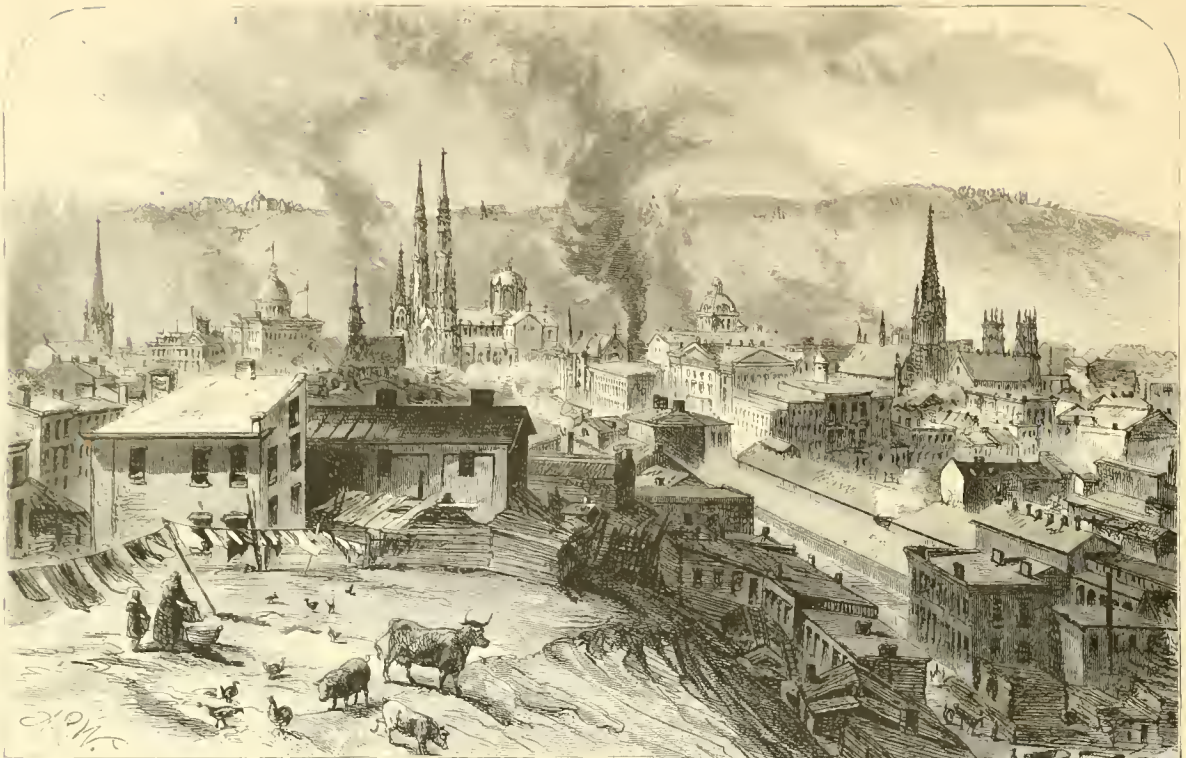
Pittsburg, from Reservoir
